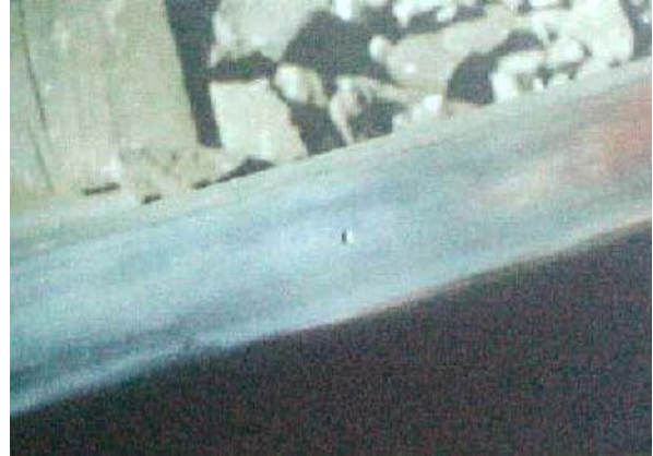
FIG. 48 : 301 - DAMAGE TO RAIL BY BRUSHING OR ARCING
